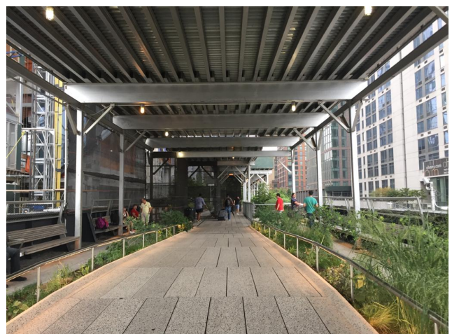
Photo 2. Smooth concrete tiles and mild slope.
